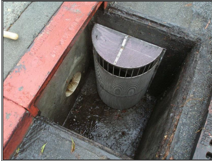
Figure 1.2. Example small full-capture device used as a monitoring site.
